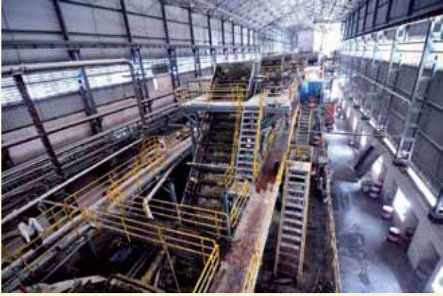
Sugar mill carrier- internal view
