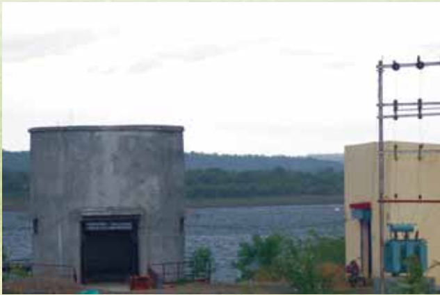
Masoli dam with Jackwell
